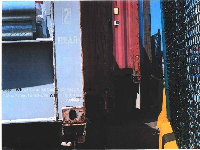
Photograph Number 3: Install Wheel Stops at Pier 3 Container Yard along Kuhio Street fence line, near water tank area
